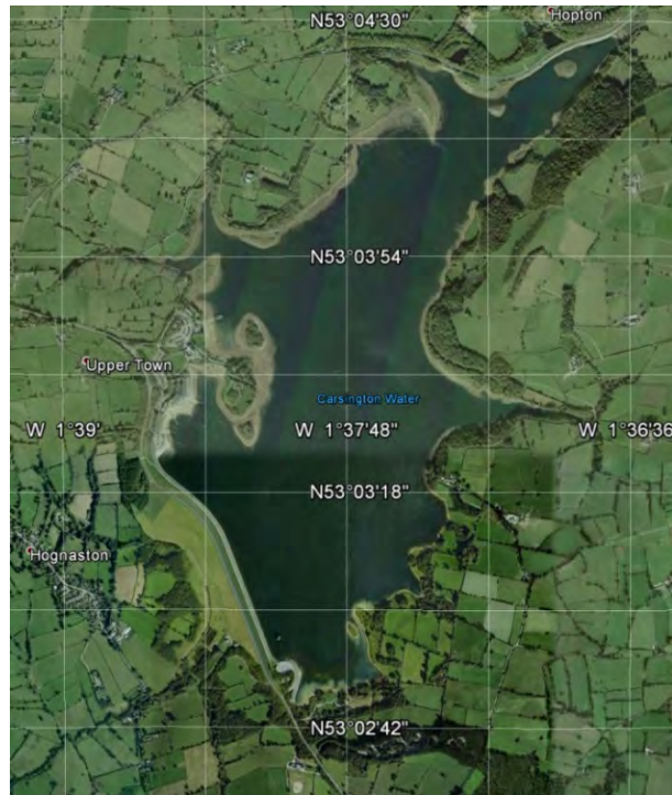
Figure 1: The study area of the Carsington Earth Embankment Dam in Derbyshire region, UK
