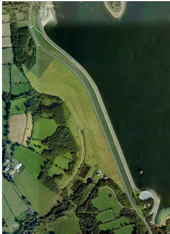
Figure 2: Close up of the reconstructed Carsington Earth Embankment Dam area.
