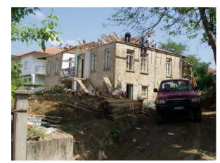
Structural rehabilitation of an old residential traditional stone building, protected by law, to a luxury hotel using irreversible and ecological solutions such as an interior steel skeleton supporting elastically the parametrical stone walls. The building is in a highly traditional protected area.
