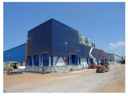
Structural optimization, final design and constructional detailing of steel industrial building with 40.0m span and 110.0m long, used as paper factory, with additional external 200m<sup>2</sup> offices for *SalcoPaper S.A.* company in Sindos, Thessaloniki, Greece.
