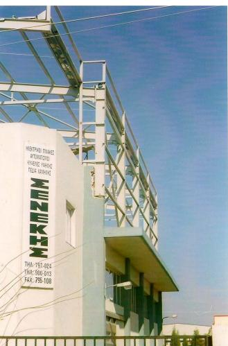
Structural design of an industrial steel building of about 1.200m<sup>2</sup> with 10 ton capacity traveling cranes and about 200m<sup>2</sup> interior office spaces for *Frost L.t.d.* in Sindos, Thessaloniki, Greece.
