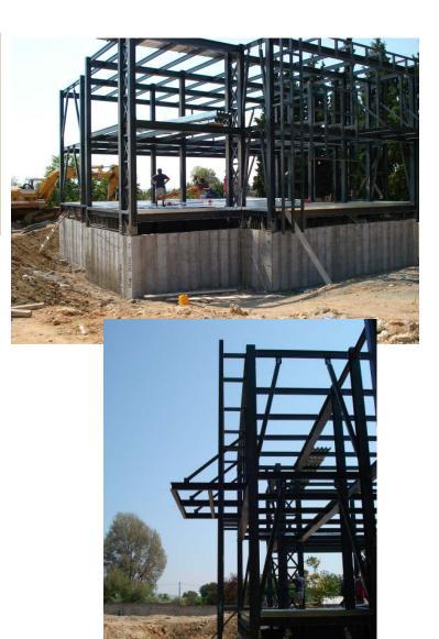
Constructional design, detailing and supervision of a composite steel-concrete 3 story residential building with pilotis, and basement, in Polichni region of Thessaloniki, Greece.
