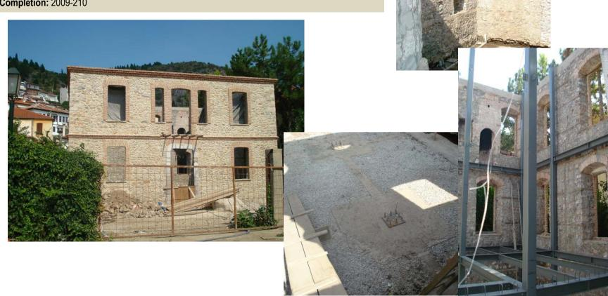
The project rehabilitation consists of structural plan, which considers the strengthening of the basement, ground floor and upper floors. The intervention consists in using four steel tubes in order to carry out the seismic actions. In the same time, by bracing the timber floors, rigid horizontal diaphragms were created.
