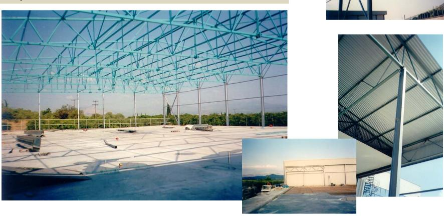
Structural evaluation of the existing building, design of a new steel roof as well as design of a steel story addition of approx. 200 m² based on a strengthened story of an existing reinforced concrete structure for *Nikolaidis L.t.d.* in Ioannina, Greece.
