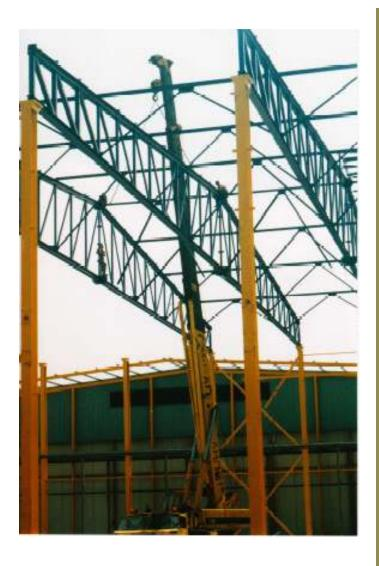
Structural cost estimation, preliminary, final structural design and constructional detailing of steel industrial facility, used as logistics center of fruits and vegetables, of 10.000m<sup>2</sup> with interior spaces of 950 m<sup>2</sup> offices, 1500m<sup>2</sup> electromechanical corridors and 500m<sup>2</sup> machine rooms for *Limpantsis S.A.* in Mesovouni, Thiba, Greece.
