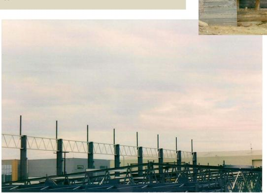
Structural assessment of an existing reinforced concrete structure and design of a new steel building 16.0m by 54.0m on the reinforced concrete structure for *Senekis L.t.d.* in Sindos, Thessaloniki, Greece.
