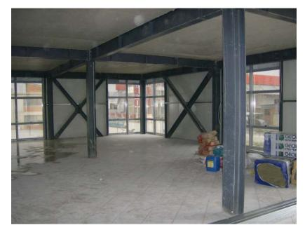
• Structural design of a new two story parking building developed on a grid of 8.0\*8.0m of about 1.200m<sup>2</sup> area with two stories of steel structure and another one story, at the basement, from steel embedded in reinforced concrete.
