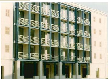
The complex is composed by 5 buildings, (3 finished at present moment). Each building has Basement (used for garage)+Ground Floor+Mezanin+5 Stories plus Penthouse. The structure is composed by composite steel-concrete frames, with a central reinforced concrete tube. The composite beams are constructed by reinforced concrete plates and castellated beams with circular openings
