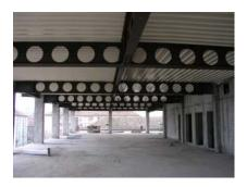
Constructional design, detailing and supervision of a steel suspended structure from an rc floor creating an intermediary space of about 1000m<sup>2</sup>. All the structure is suspended from the reinforced concrete plate, existing rc columns and some parametrical rc walls.
