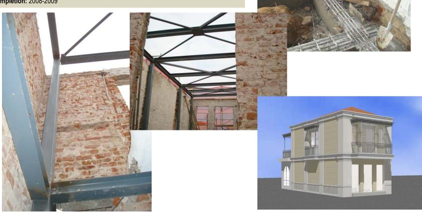
Structural rehabilitation of an old residential traditional stone building protected by law, using irreversible and ecological solutions such as steel, wood and stone elements.
