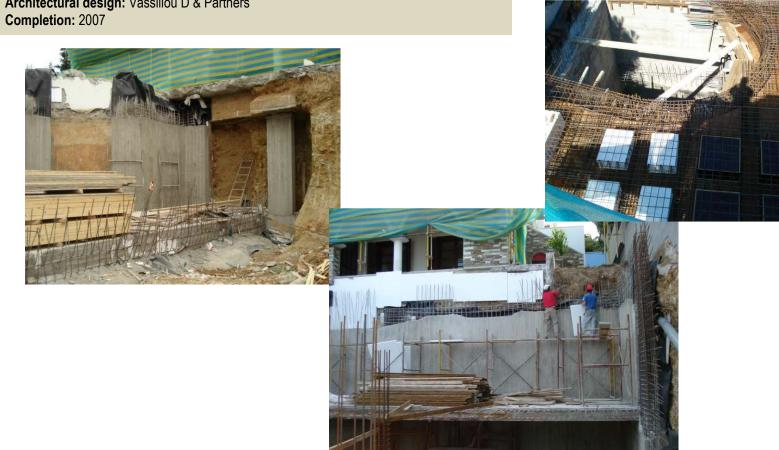
Structural rehabilitation of an old residential building constructed in 1925, protected by law, to a new small office consecrating the exterior shell and developing a new steel structure which support elastically the exterior façade.
